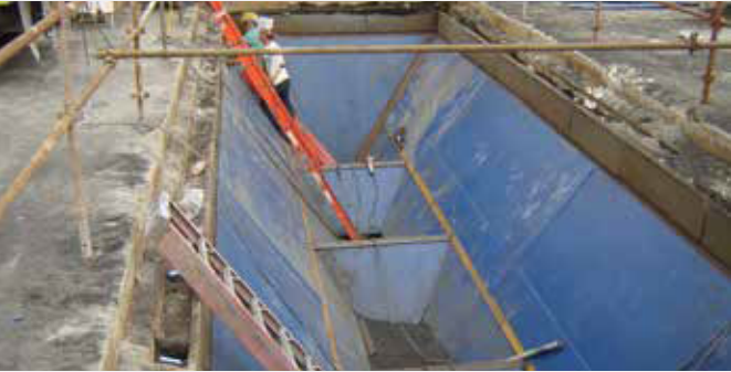
Four outlet phosphate receiving hopper lined with TIVAR® 88-2
